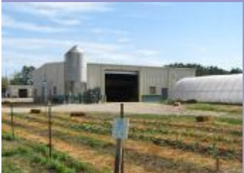
The Agriscience barn construction was completed for the 2007 school year.
